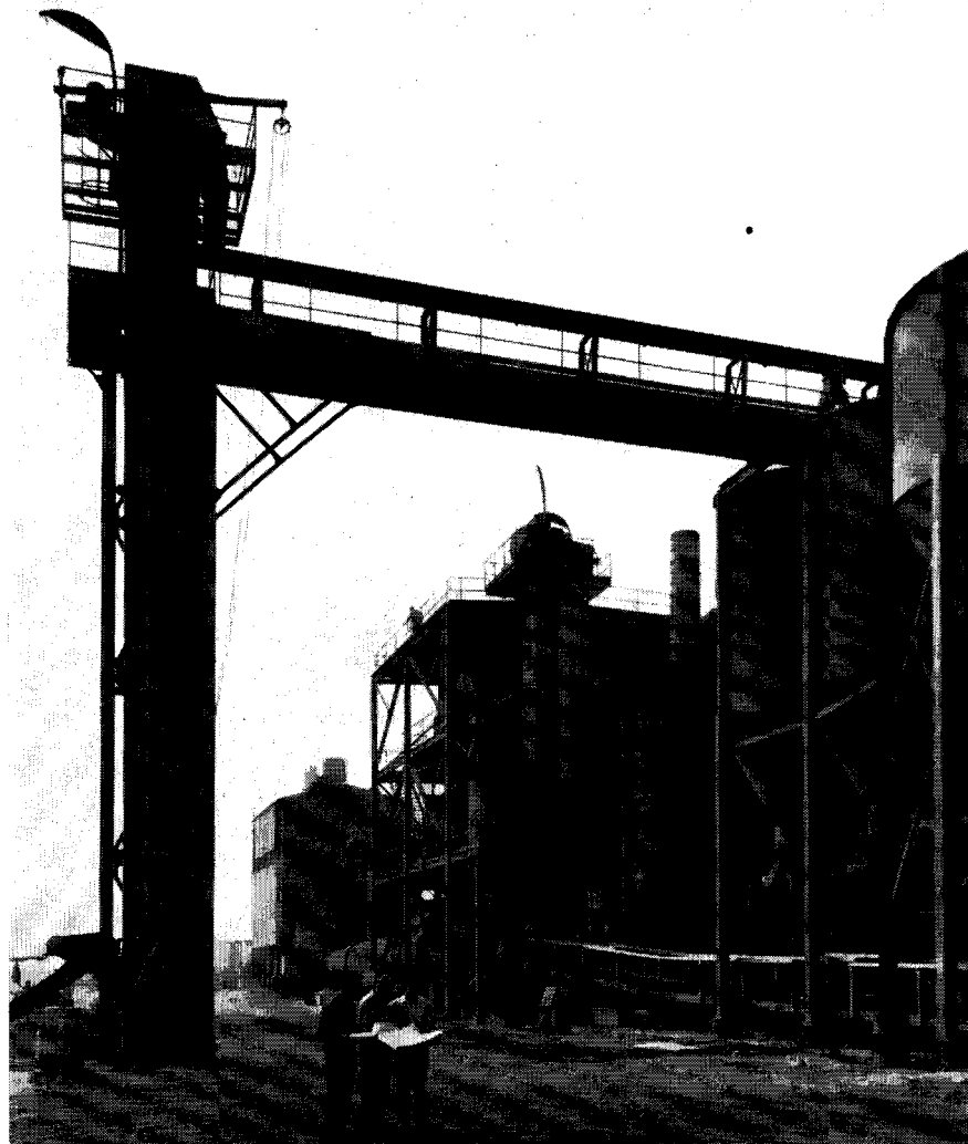
Before year's end, pelletized 17-7-0, 10-10-10, 10-10-5, and 5-15-0 will be coming from this Stauffer unit at Vernon, Calif. Manufacturing Section (center) includes pelletizers, grinders, weighers. Raw material bins at right
